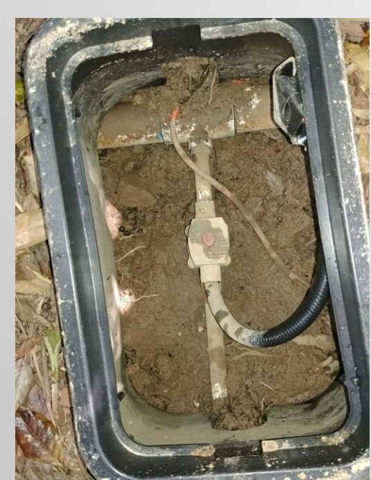
Automated valve timed to drain storage tank every 7 days
