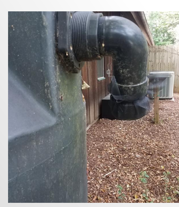
Screening and sealing all potential entries to internal part of the tank
