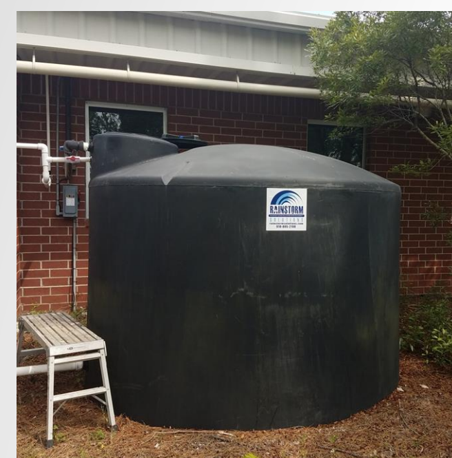
Rainwater harvesting system
