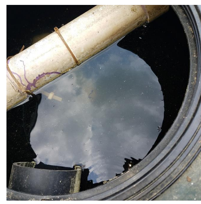
Standing water inside RWH storage tank
